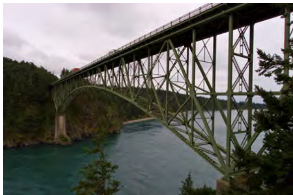
1 - Diablo Lake, North Cascades National Park 2 - CCC Picnic Shelter, Bowman Bay 3 - Deception Pass State Park 4 - Deception Pass Steel Bridge
